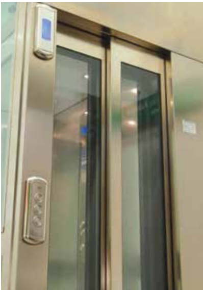
Car and landing door with framed glass "big vision" type
