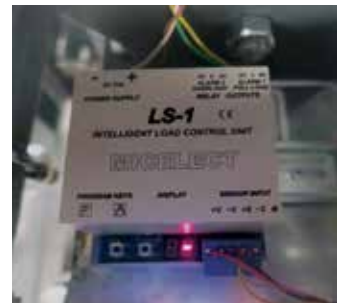
Car load weighing device (standard for 100 ONE and Double Decker models)
