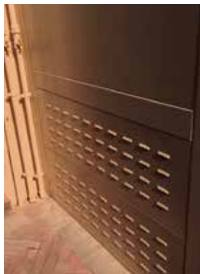
Steel plate cladding with aeration slits
