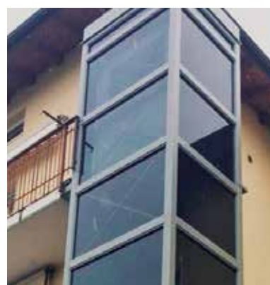
Reinforcement cross-braces for headroom without anchoring points
