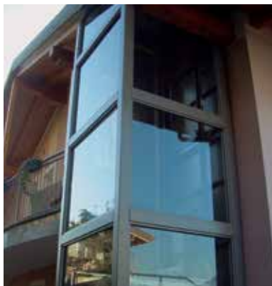
Glass holding profiles and gasket for structure EXTERNAL face installation
