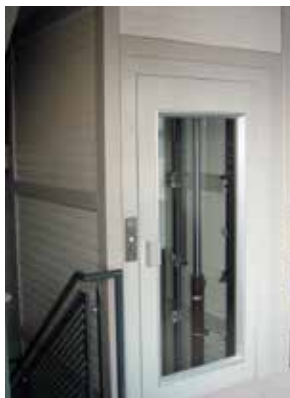
Cladding with sandwiched insulating panels RAL 9002
