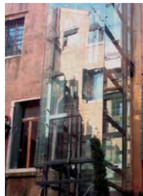
Cladding with outer structure glass and stainless steel fixing studs
