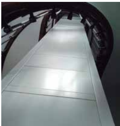
Baked enamel RAL steel plate cladding, stainless steel or skinplate
