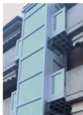
Gangway connecting structure to the building
