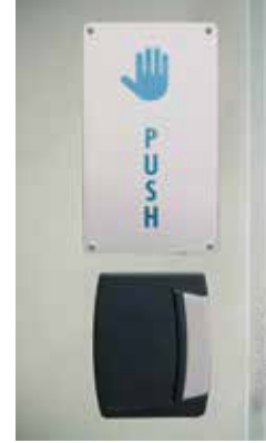
Landing door internal closure handle
